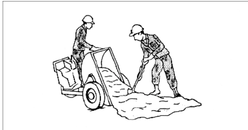
Figure 5-8. Handling concrete by power buggy
